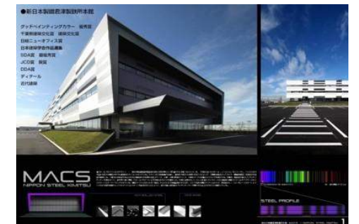
●NIPPON STEEL KIMITSU MAIN BUILDING (Kimitsu City, 2011)
