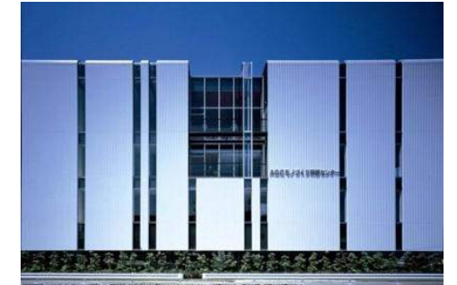
●AGC MONOZUKURI TRAINING CENTER (Yokohama City, 2006)
